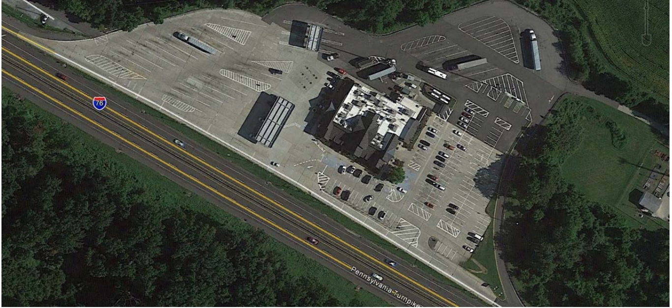
Figure 10: Peter J. Camiel Service Plaza - Milepost 304.8 Westbound
